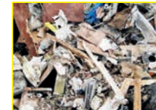
CONSTRUCTIONS & DEMOLITIONS SORTING HEAVY FROM LIGHT MATERIALS
